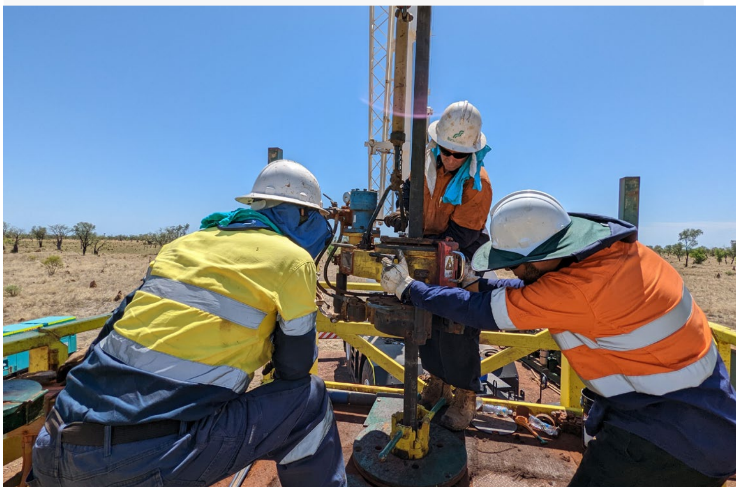
Well decommissioning operations
