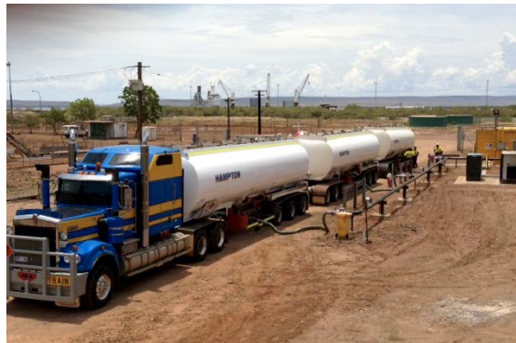
Offloading at Wyndham storage facility
