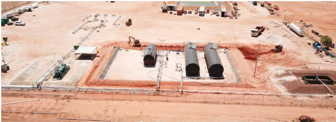
Ungani Facility tank upgrades
