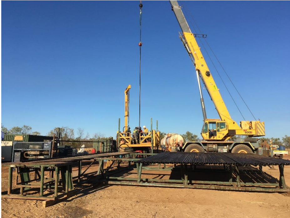
Buru Jacking Platform operations on Lennard Shelf well
