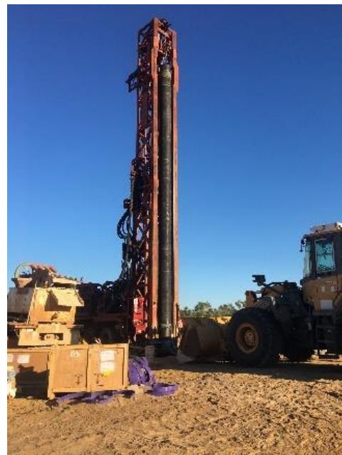
Installation of 20 inch drilling conductor
