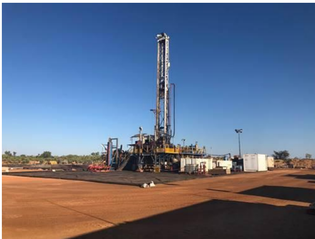
DDGT1 Rig on Ungani 4ST1 well location
