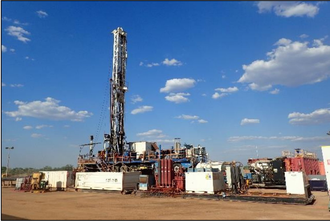
DDGT1 Rig on Ungani 4 well location
