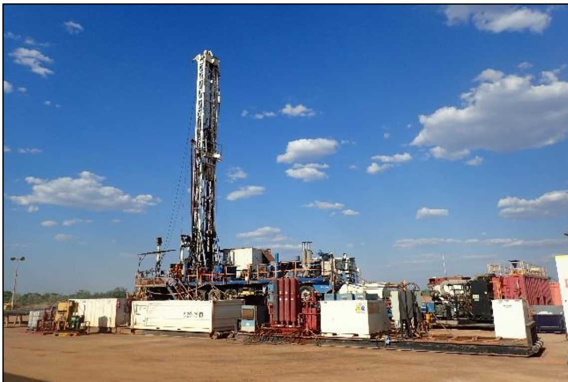
DDGT1 Rig on Ungani 4 well location
