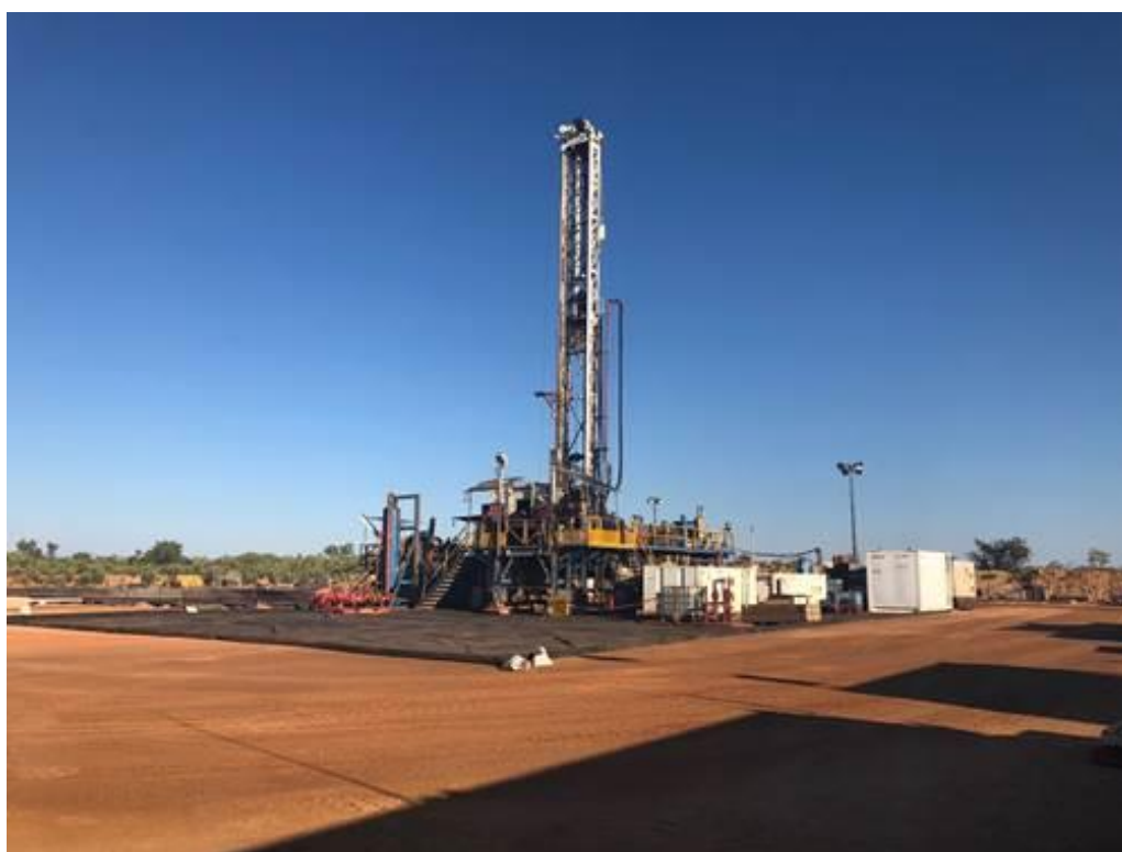
DDGT1 Rig on Ungani 4ST1 well location
