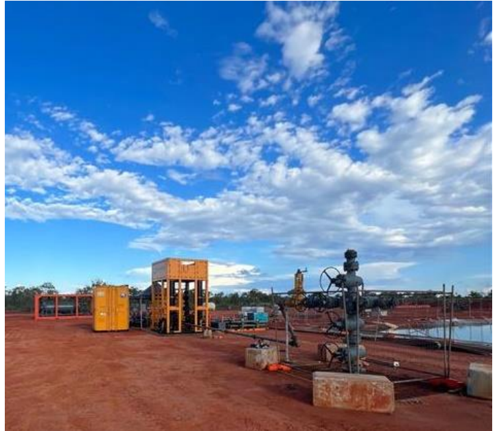
Testing equipment at the Rafael 1 well site
