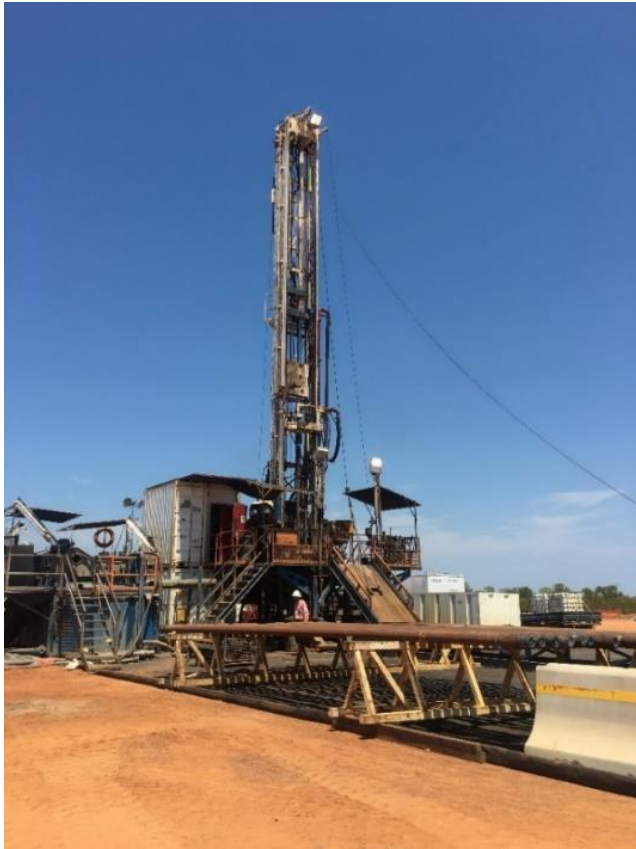
DDGT1 Rig on Ungani 5 well location
