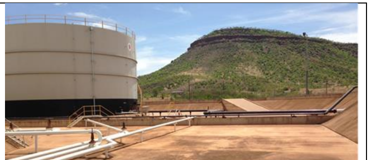
Wyndham Tank Farm and Piping Modifications
