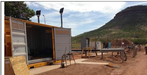
Wyndham Truck Unloading Bay
