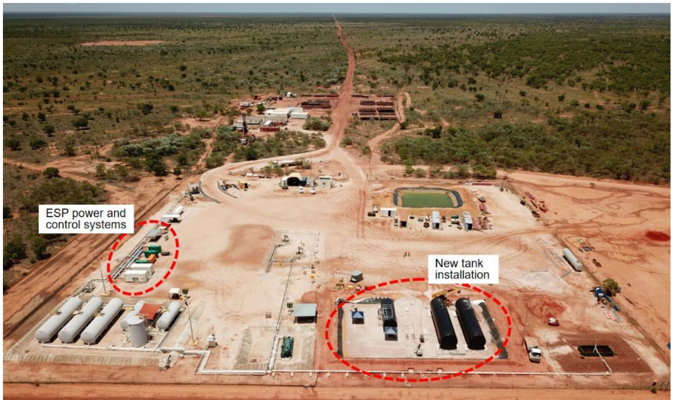
Ungani Production Facility showing ESP surface equipment and new tank installation
