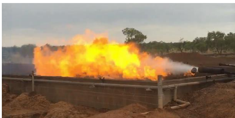
Valhalla North cleanup flow (8 January 2016)
