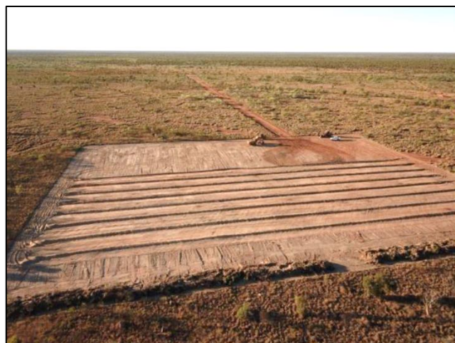
Ungani West 1 site clearance
