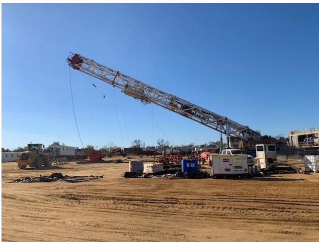
Rigging down at Currajong 1
