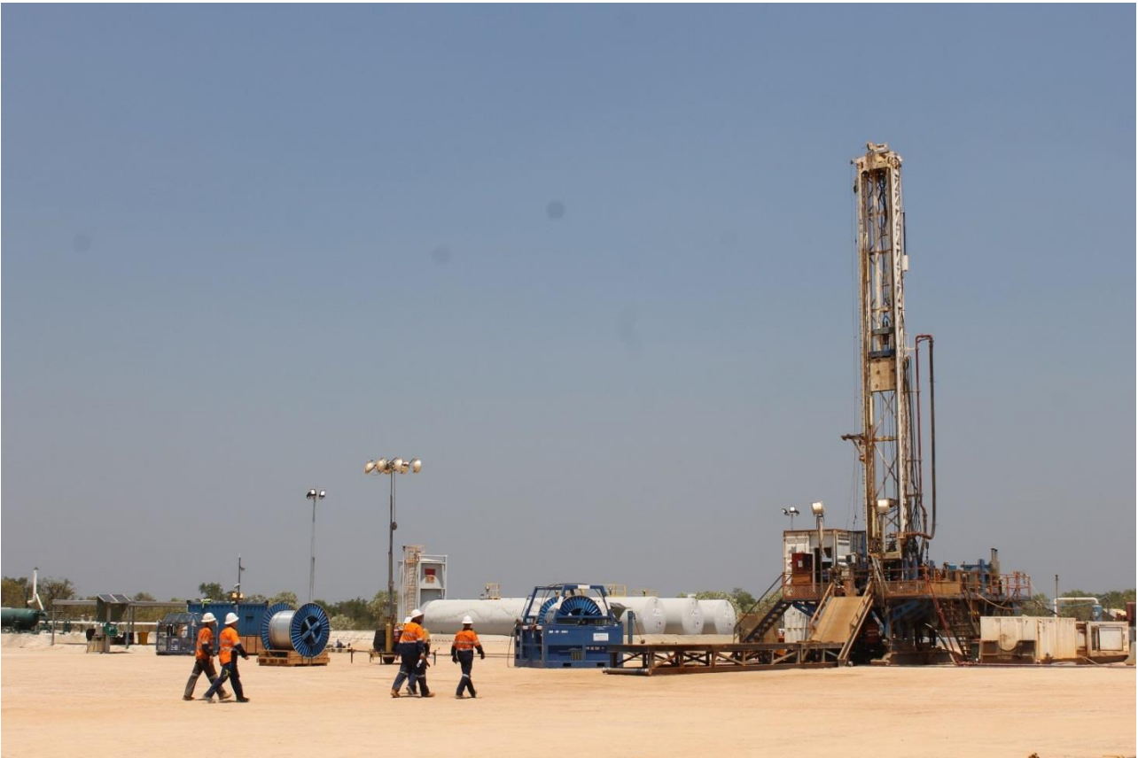
DDGT1 rig on the Ungani 1ST1 well site
