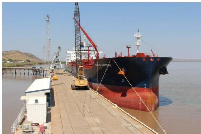
Ship loading at Wyndham
