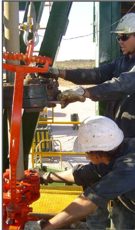
Drilling operations on the Fairway Rig
