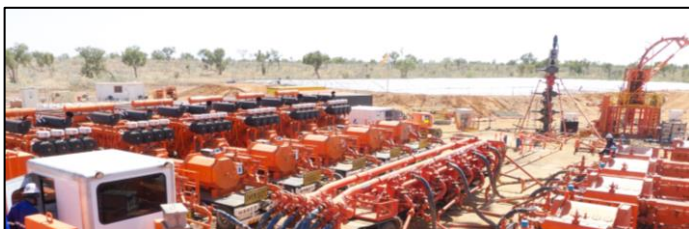
Condor Energy on location at Asgard 1 well site on Noonkanbah station.
