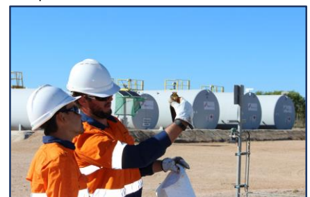
Ungani Production Facility
